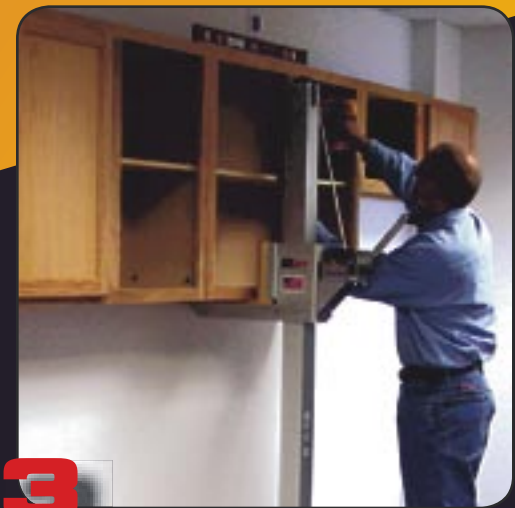
Raise cabinet to desired height and mount on the wall.
