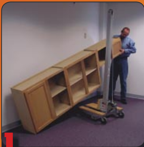
Load upper by lifting one end and rolling lift under.
