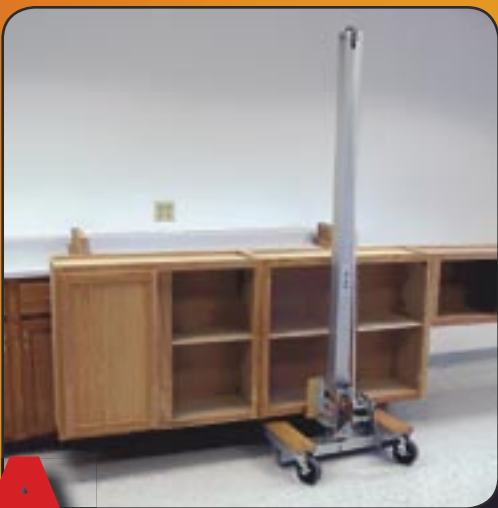
Position loaded upper in front of base.
