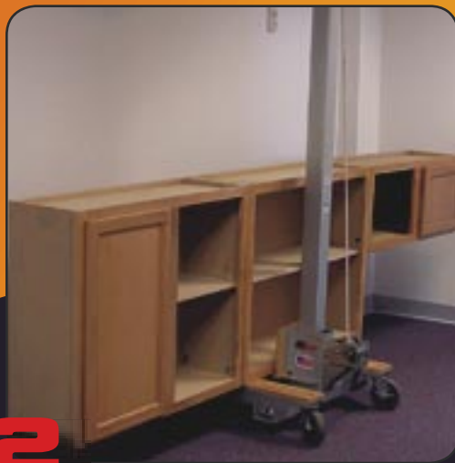
Balance cabinet on lift and position in front of wall.
